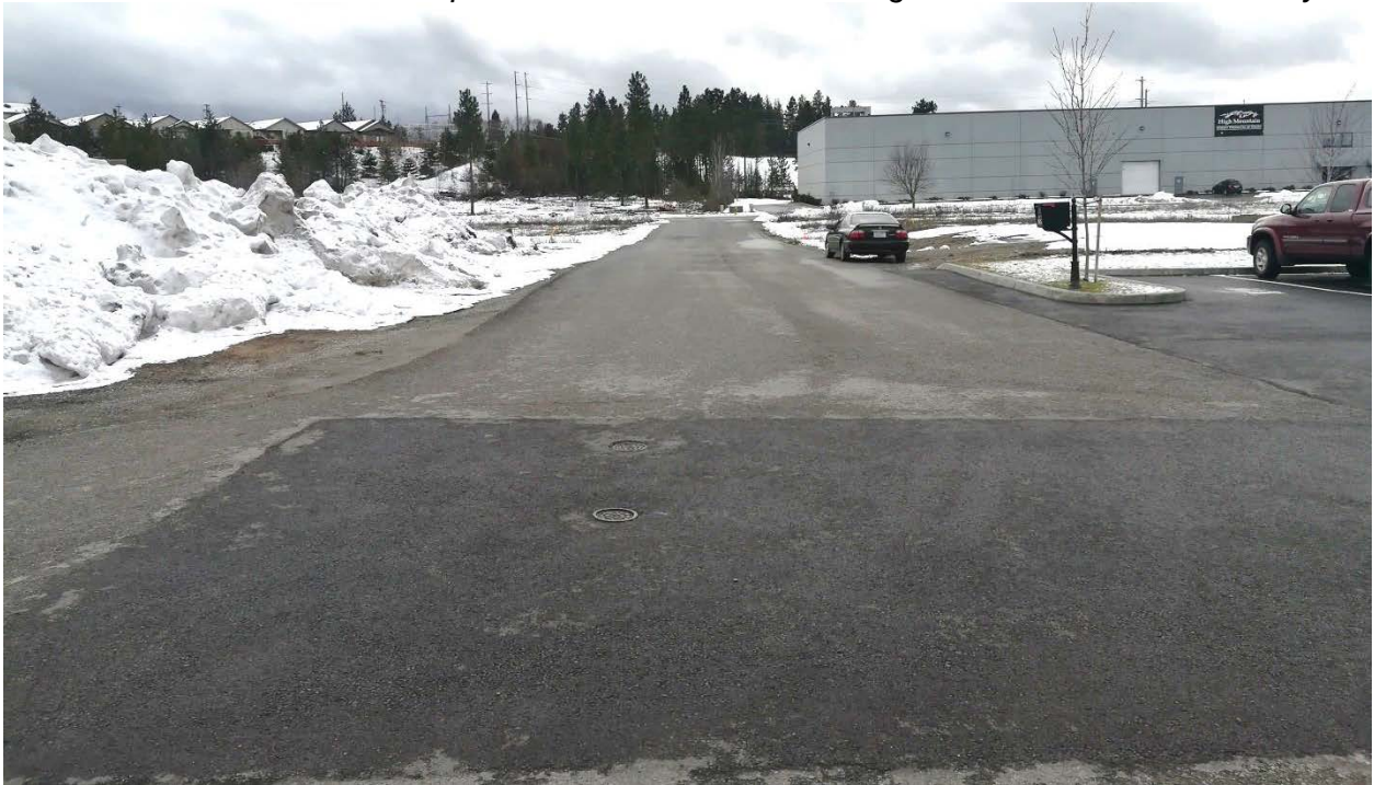
Internal paved access to the site looking south toward Schreiber Way:
