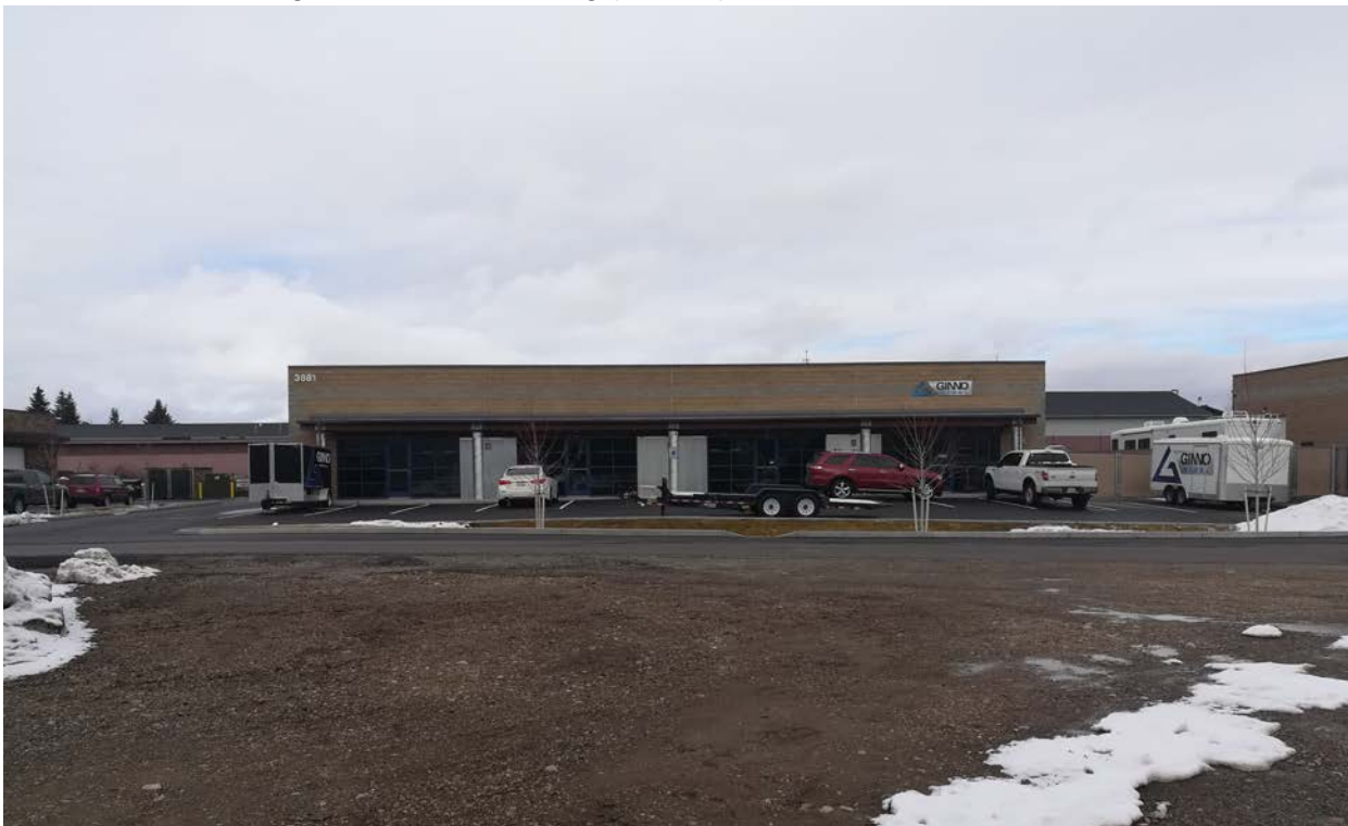
Existing multi-tenant building (Site #2):
